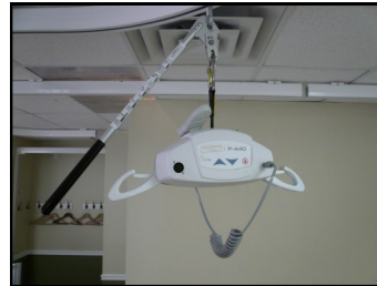
Figure 9A - Photo showing P-440 lift carabiner connected to a reacher first and then to the eyelet of the trolley.
