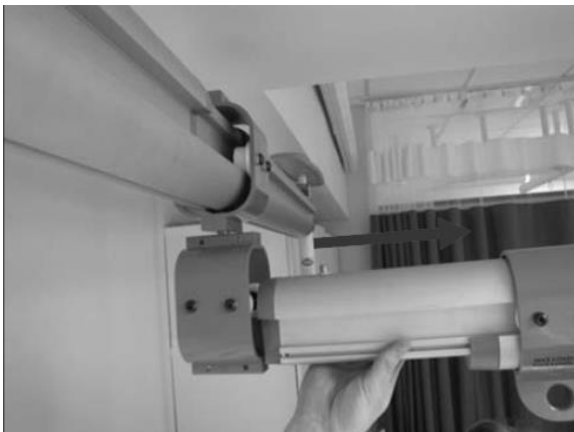
Figure 31: Remove the Traverse Track from the Trolley
